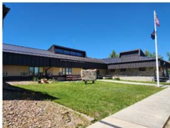
Front of Hospital
